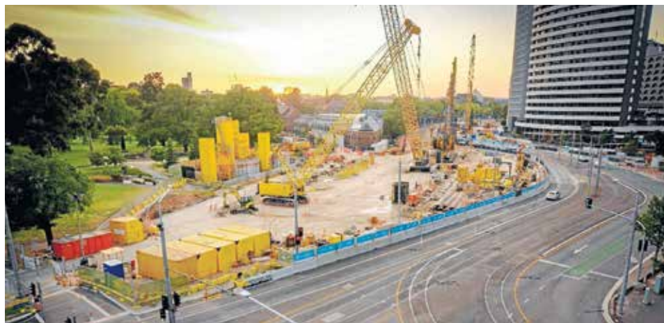
▲ The ANZAC station worksite at St Kilda Rd.
