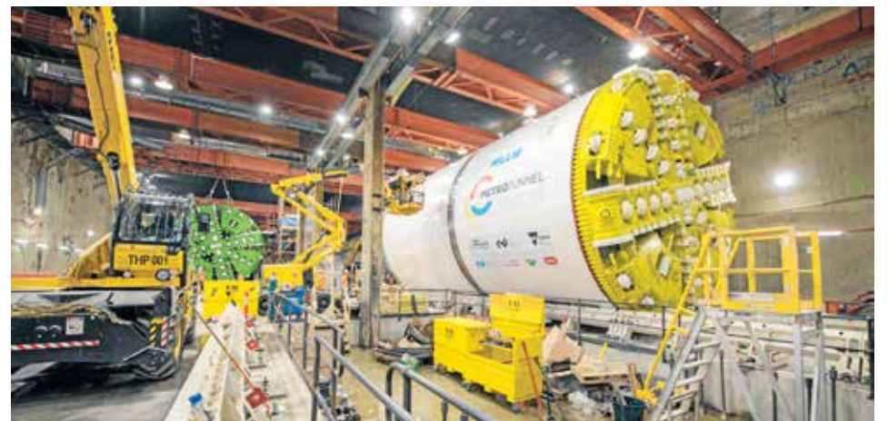
▲ Tunnel Boring Machines underneath St Kilda Rd.
