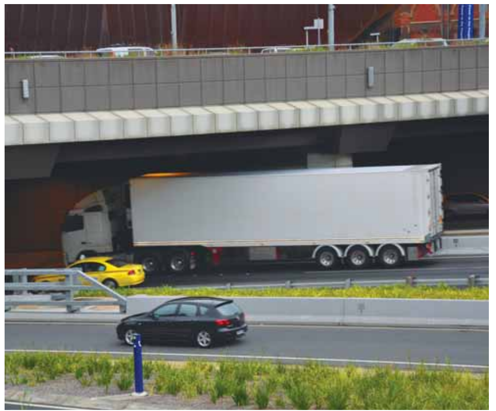
Trucks entering the Burnley Tunnel will now need to ensure they are not making too much noise.
