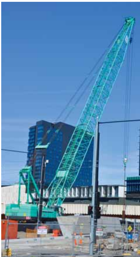
Work is nearing completion on the Jim Stynes bridge.
