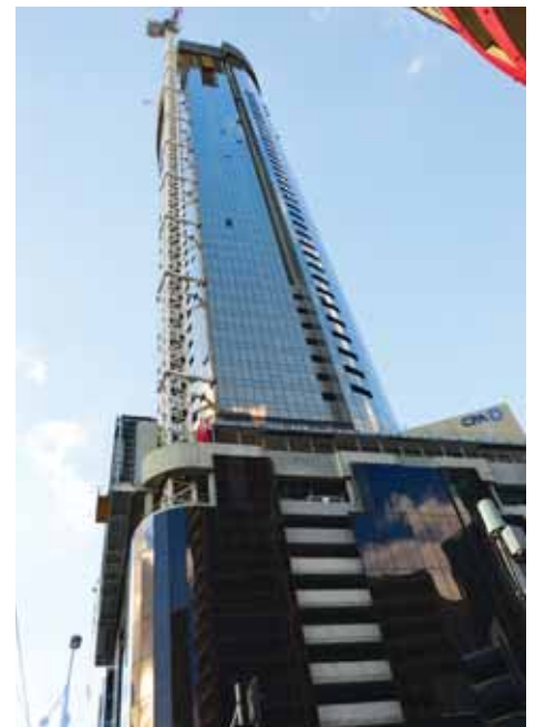
Prima Pearl tower in Southbank.
