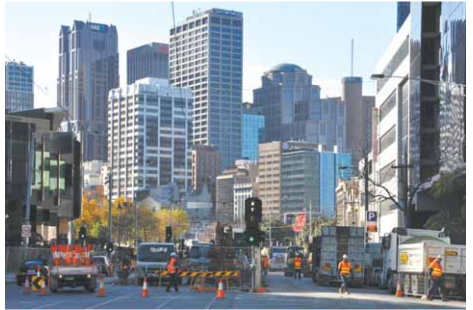
Queensbridge St during last month's tram network construction works.
