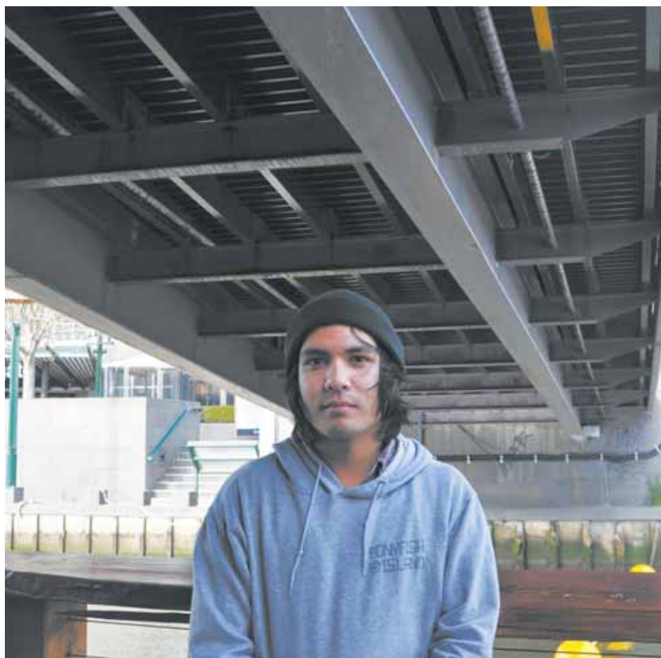
Ponyfish Island bar manager Thomas Auer said the noise from the bridge's new decking was upsetting his customers.
