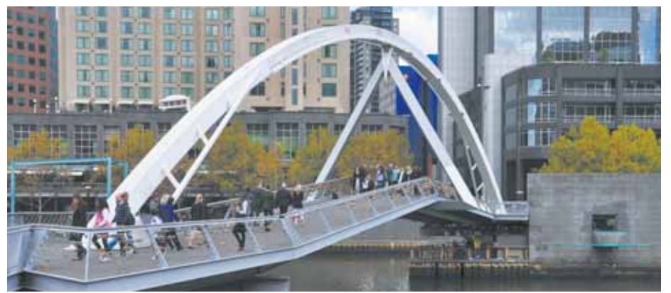
The Southbank Footbridge has officially been renamed the Evan Walker Bridge.
