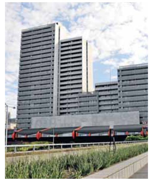
The Guild apartments on Sturt St, Southbank.
