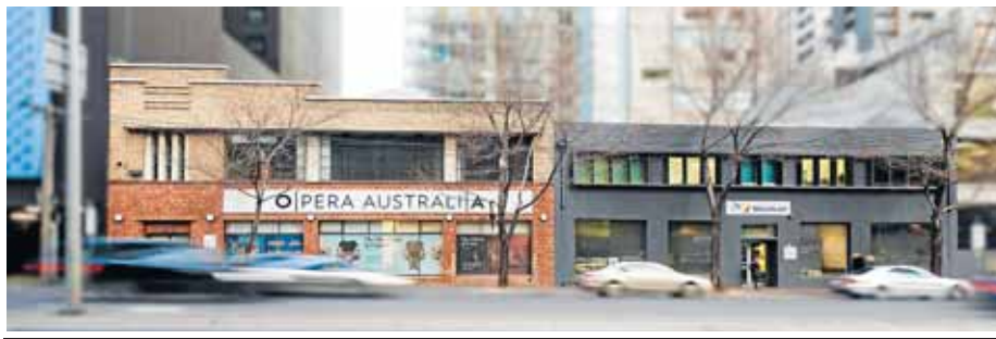
The dual development site at 35-41 and 43-47 City Rd.
