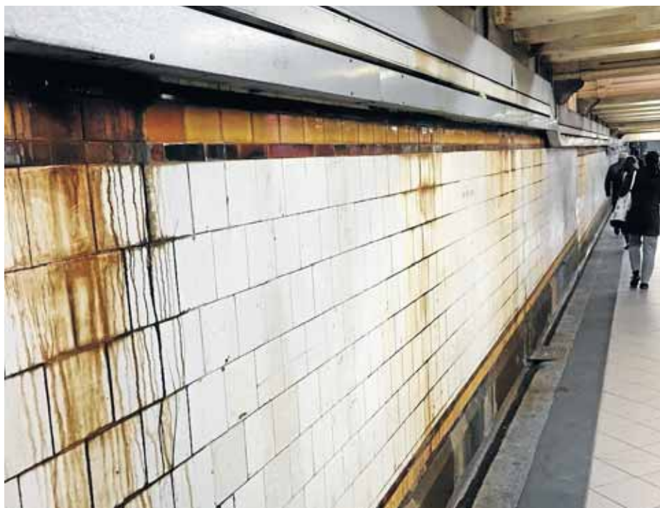
The Elizabeth St underpass at Flinders Street Station.
