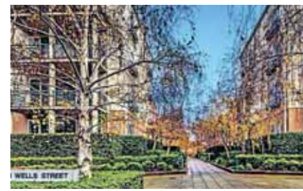
The Keep Apartments at 88 Wells St.
