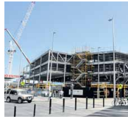
The construction site at South Wharf.
