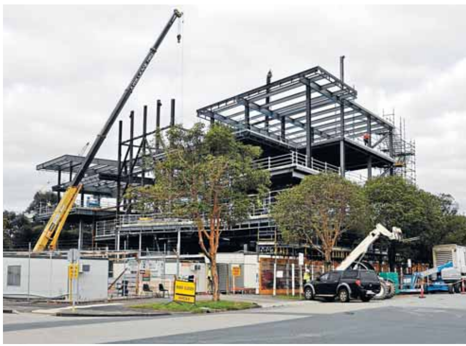
Southbank's new primary school on Ferrars St is quickly taking shape.
