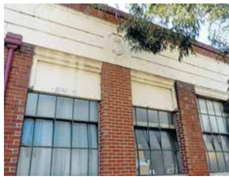
The site of the former General Post Office in Sturt St.
