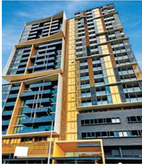
The Guilfoyle is a Southbank apartment complex understood to have cladding concerns.
