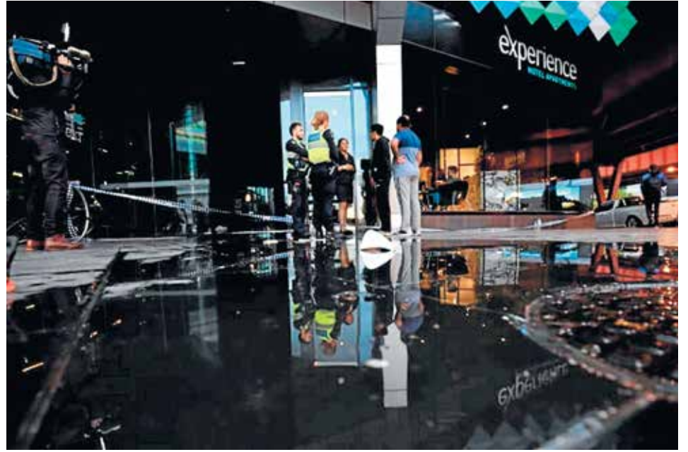
Experience Bella Apartment tower was the victim of severe flooding last month.
