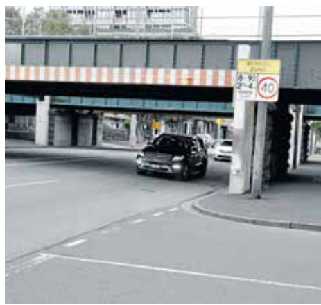
The intersection next to the Montague Street Bridge.
