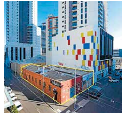
The site at 54-56 Clarke St, Southbank.
