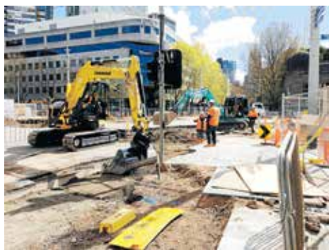
Construction of a new park at Southbank Boulevard.
