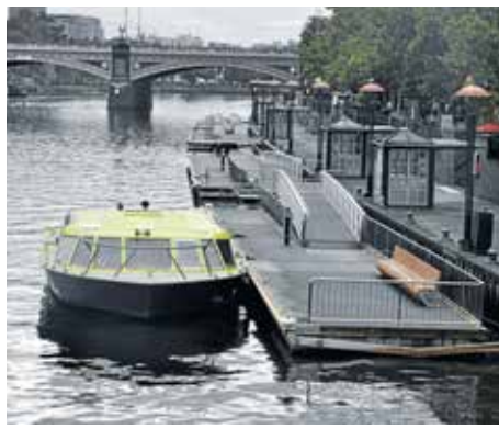
New floating berths at Southgate.
