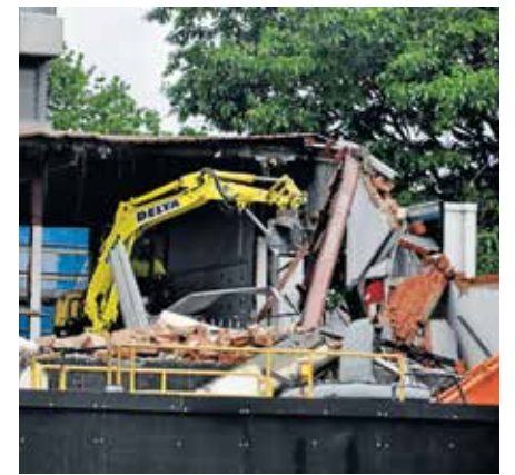
The classroom building at Boyd is demolished.
