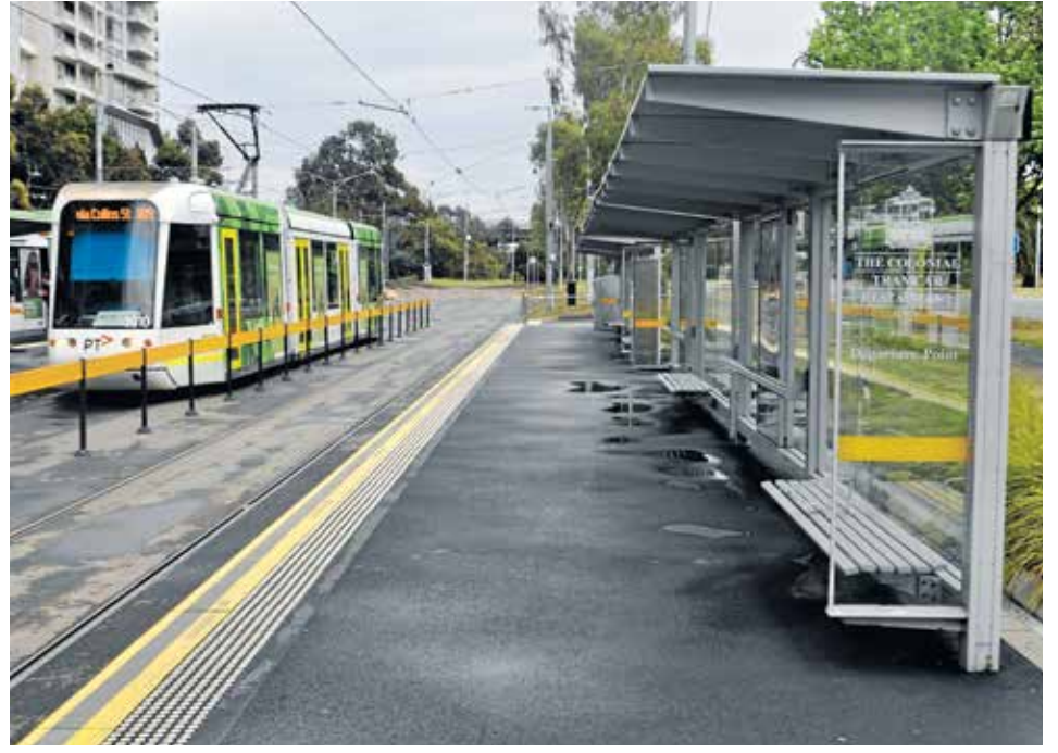
Colonial’s temporarily vacant terminal at the Whiteman St interchange, which is shared by routes 96 and 109 (left).
