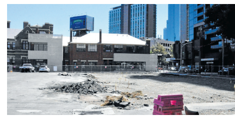
The site at Boyd Park has now been cleared.
