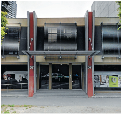
The building due for demolition at 57 Haig St.
