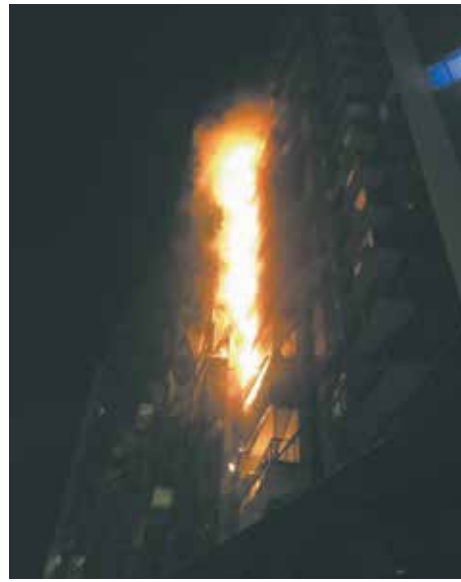
The 2014 Lacrosse building fire in Docklands triggered a national inquiry into combustible cladding.
