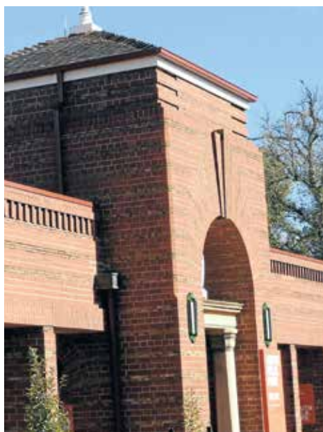
The drill hall on Albert Rd, now home to South Melbourne Park Primary School.
