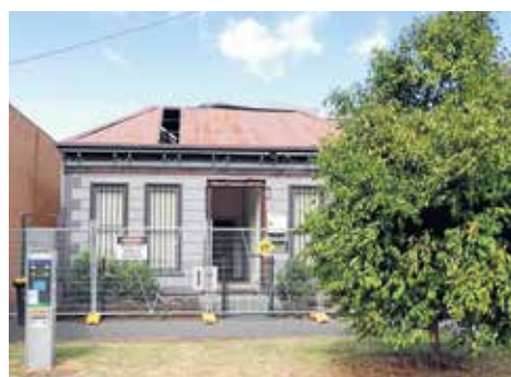
161 Buckhurst St, possibly the last double-fronted house remaining in Montague, was demolished in April.
