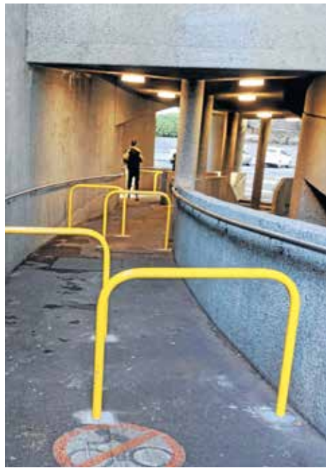
The new barriers at Hamer Hall.
