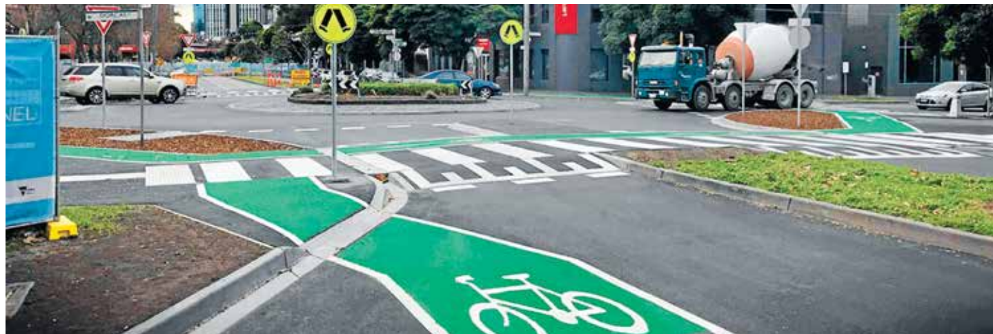
The new bike lanes on Moray St, which run from Albert Rd, South Melbourne to City Rd, Southbank.
