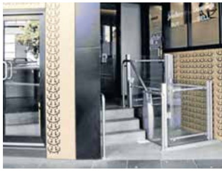
External loading lifts, like that at Banque 88 on Clarke St, are now a thing of the past under C308.
