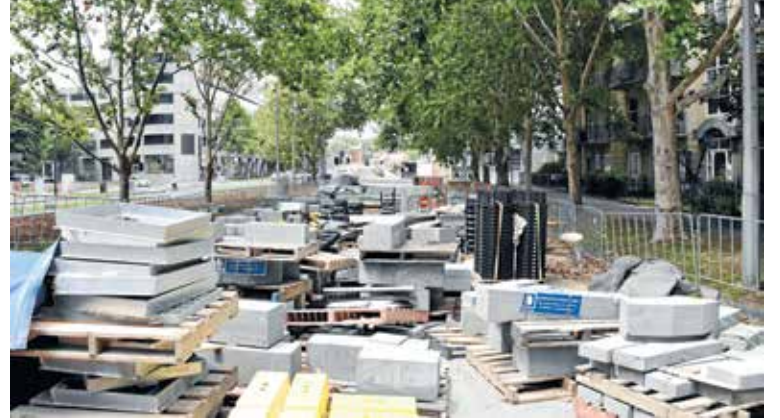
▲ Construction materials fill Southbank Boulevard between Kavanagh and Moore streets.
