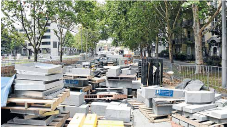
▲ Construction materials fill Southbank Boulevard between Kavanagh and Moore streets.
