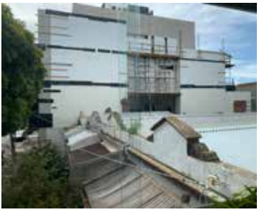
▼ Single family home, another two storeys to be built, Gladstone St.
