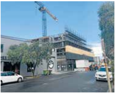
▼ Towers in Thistlethwaite St under construction
