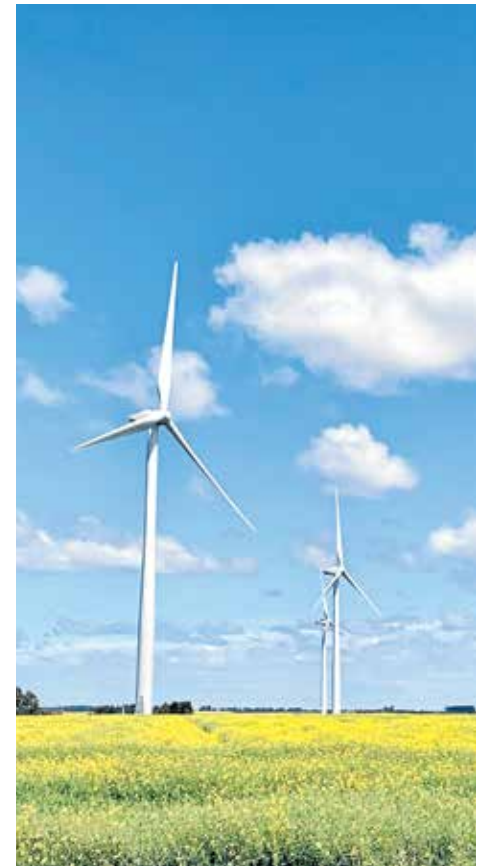
▲ Yaloak South Wind Farm near Ballan.
