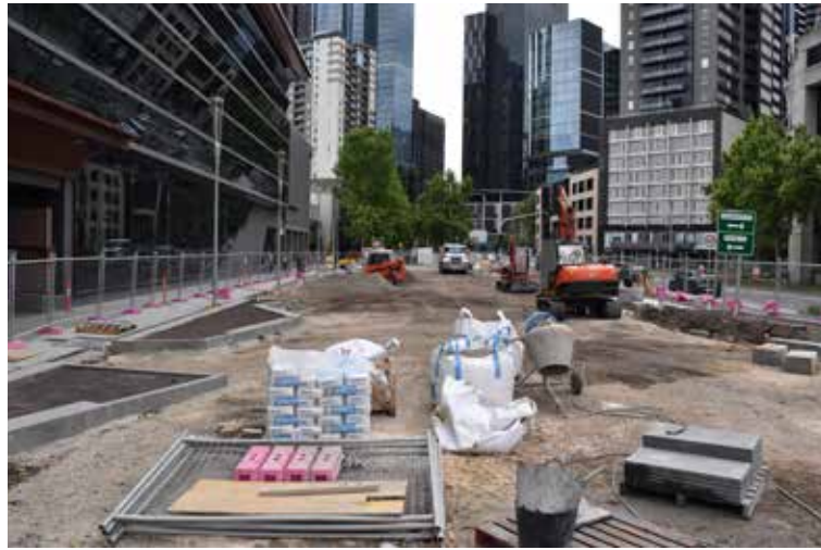
▲ Work continues outside the ABC Building on Southbank Boulevard.
