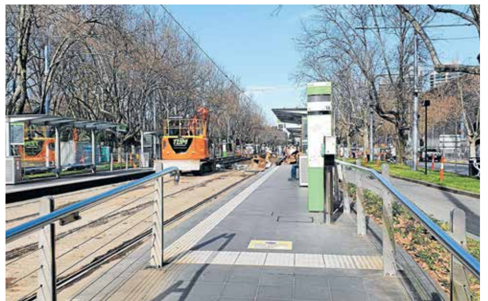
▲ Construction takes place on St Kilda Rd near Arts Centre Melbourne last month.
