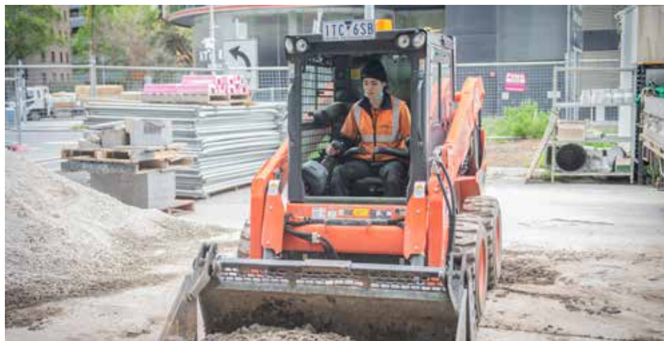
▲ Construction workers continue work on Southbank Boulevard on October 5 following the government’s shutdown.
