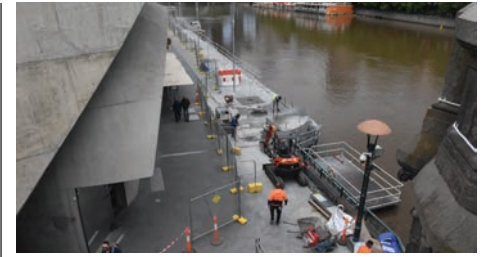
▲ View of the promenade works from Princes Bridge.
