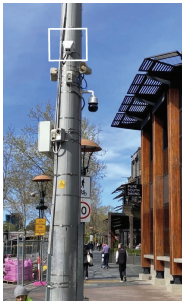
▲ The speed sensor at Southbank Promenade.
